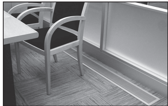
The CT-TAF-L is shown installed in a corporate office
