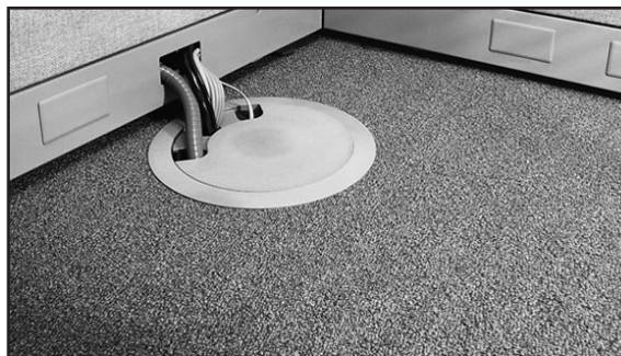
Above: Installed TAF-G in an office environment
