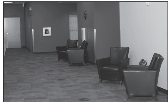
TAF-R diffusers installed in a government facility
